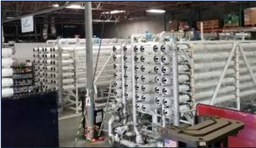
Caption: Assembly of reverse osmosis trains at Biwater Inc
